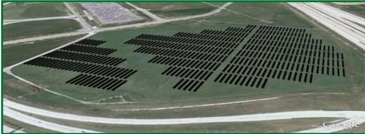
Indianapolis Airport solar farm 8
