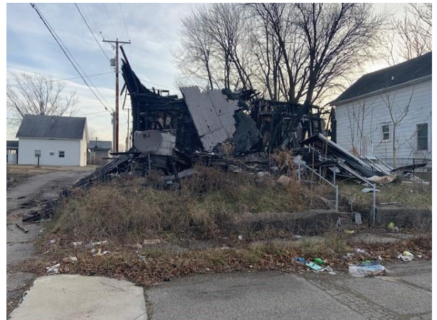
225 N. Franklin (house & garage)
