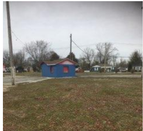
Digital photograph showing current conditions from interior field looking at the Cooley park concession and restroom building.
