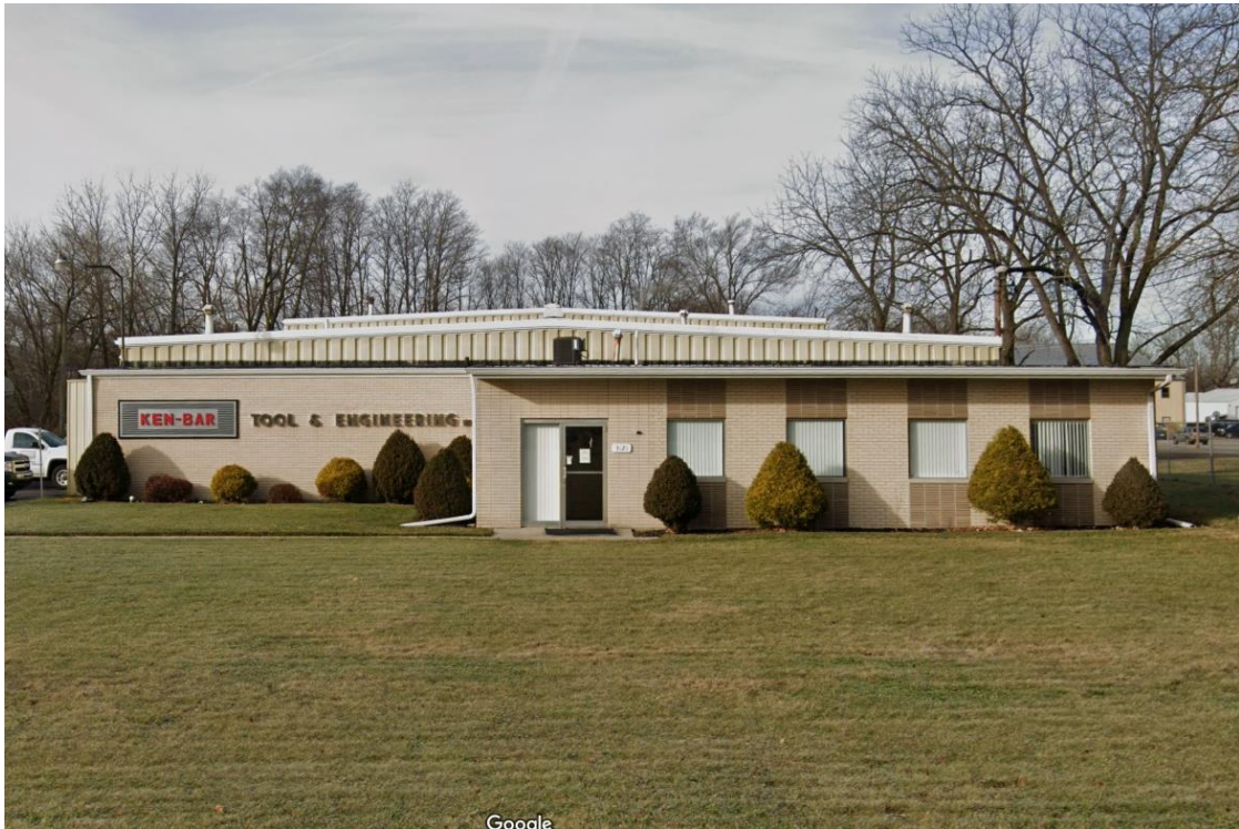
Photo 15, Camera facing W
